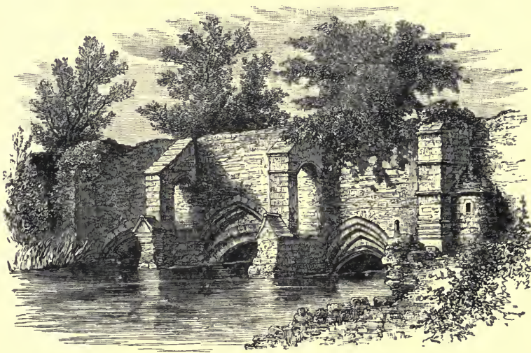
ABBOT'S BRIDGE, S. EDMUNDSBURY. Early Thirteenth Century.
